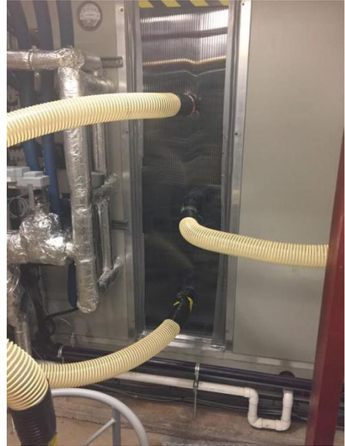
**Diagram 1.** Hydrogen Peroxide Vapour injection into the air handling unit
